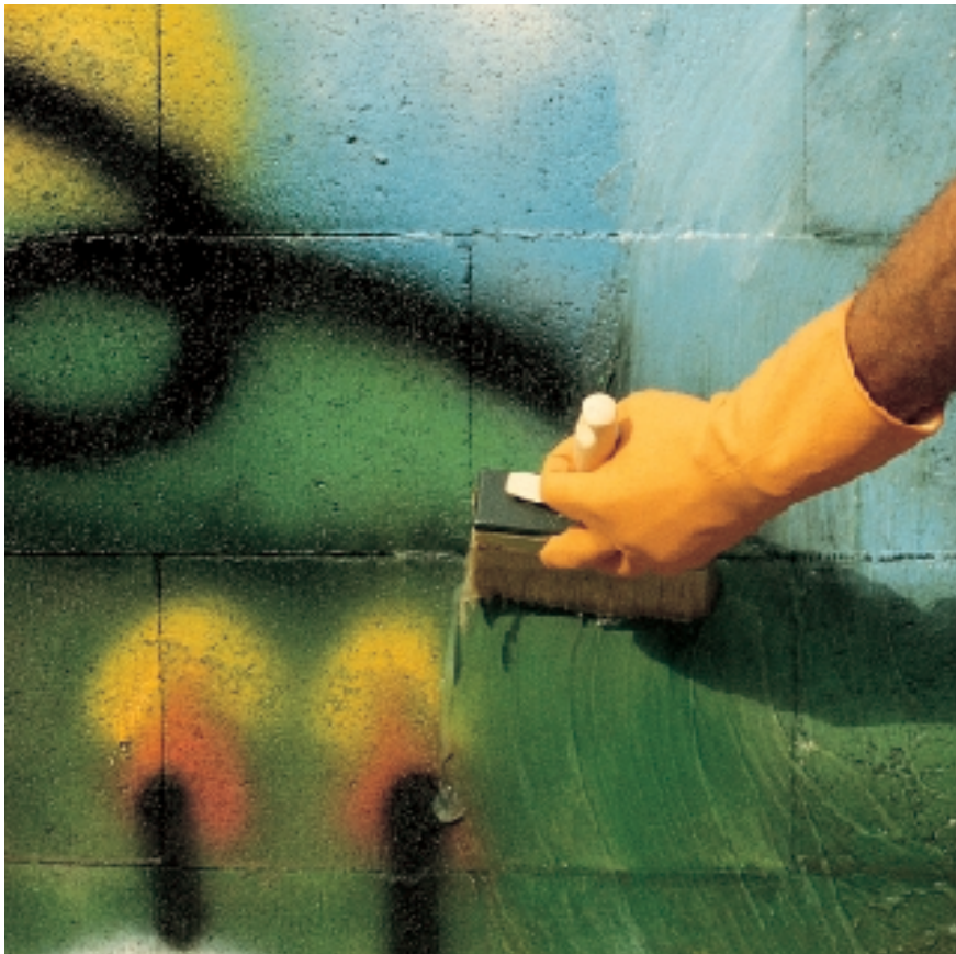
Applying WallGard GRAFFITI REMOVER GEL with a brush
