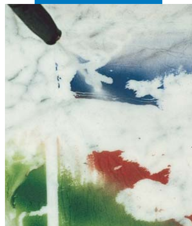
Using a high-pressure cleaner on Carrara marble treated with WallGard Graffiti Barrier
