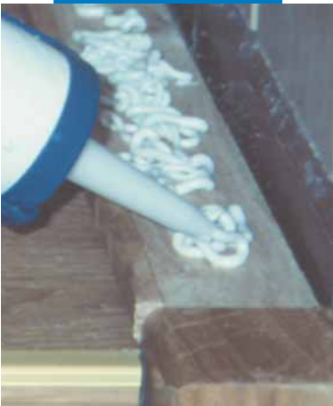
Bonding a wooden skirting with Ultrabond Eco 575
