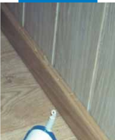
A wooden skirting applied with Ultrabond Eco 575
