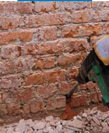
Preparing the holes in the masonry off-set from the centre
