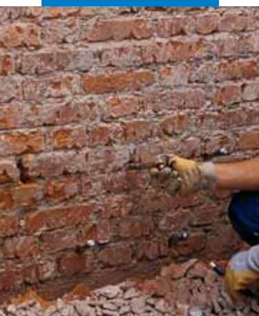
Inserting the injectors in the holes
