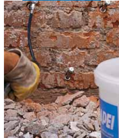
Injecting Mapestop at low pressure
