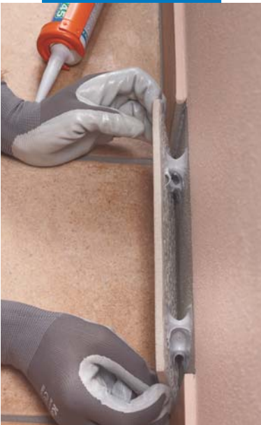
Flexible bonding of elements
