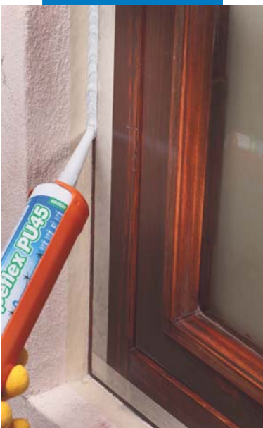
Flexible sealing of joints
