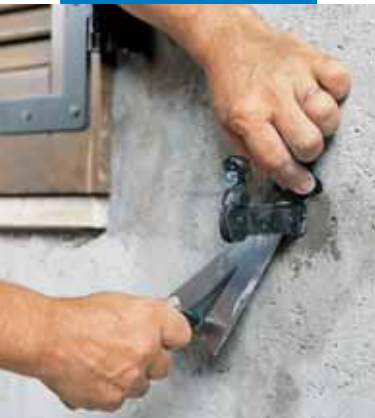
Fixing foundation bolts for windows using Lampocem
