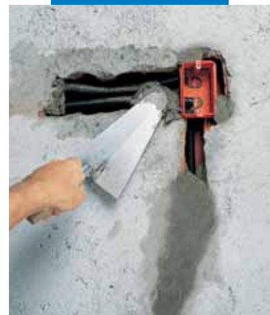
Fixing enclosures and electric cable tubes using Lampocem
