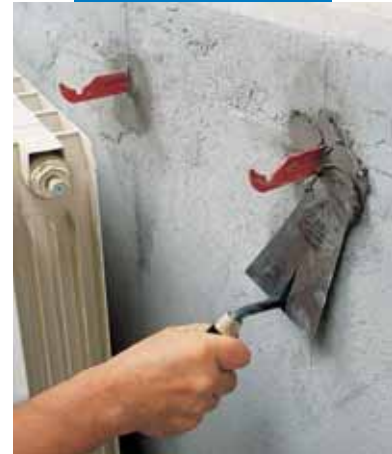
Fixing anchor bolts for radiators using Lampocem
