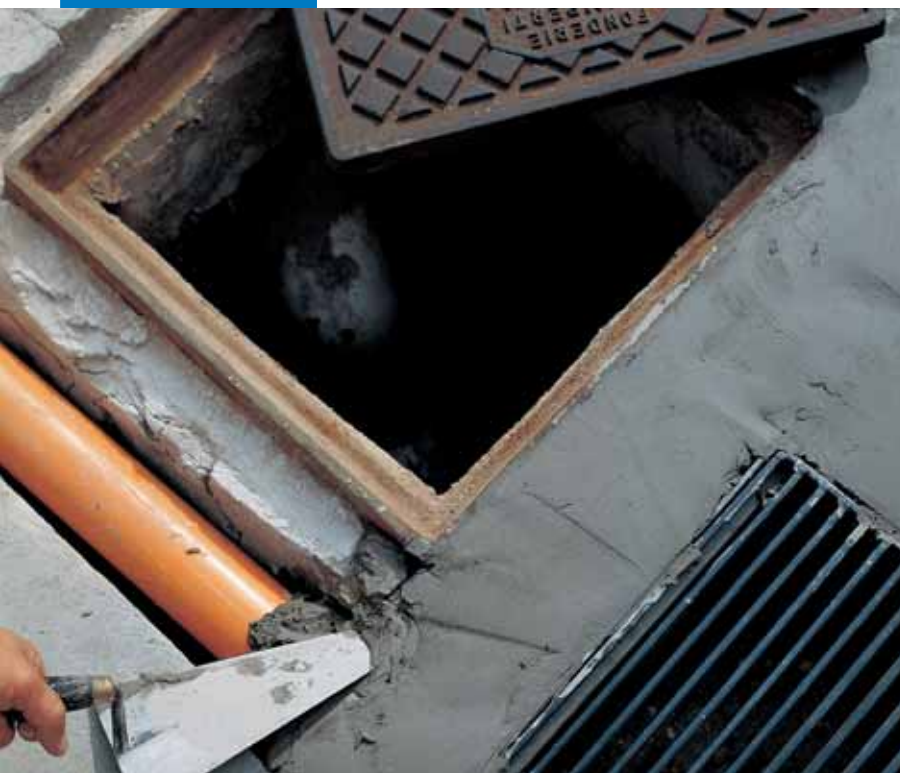
Laying pipes and manhole covers using Lampocem
