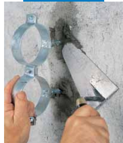
Fixing brackets for pipes using Lampocem
