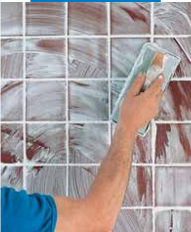
Laying the product with a rubber float
