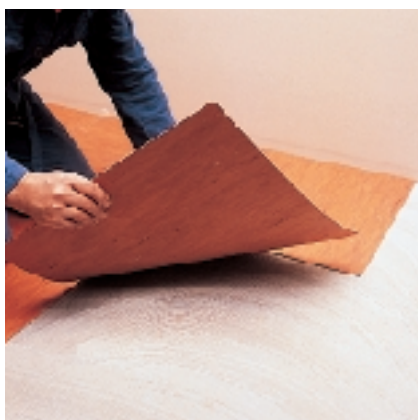
Installing homogeneous PVC tiles over ADESILEX V4
