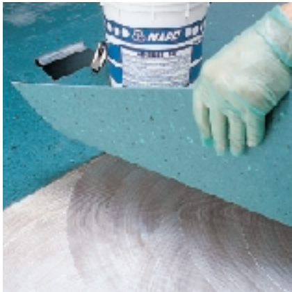
Installing homogeneous PVC tiles with ADESILEX V4, bonding on two adjoining sides
