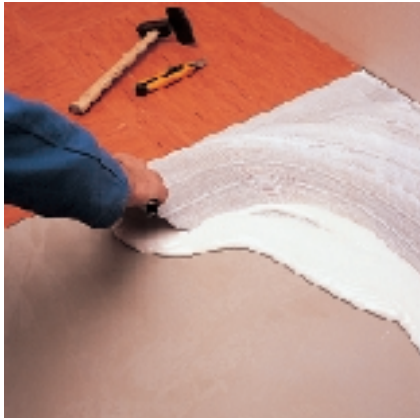
Spreading ADESILEX V4 for installation of homogeneous PVC tiles
