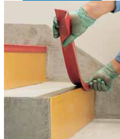
Installation of a PVC step nosing
