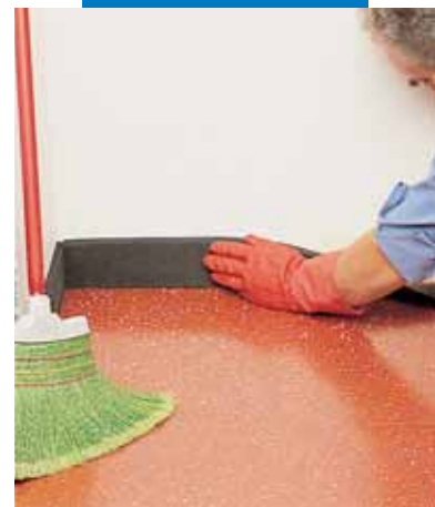
Bonding of PVC skirtings
