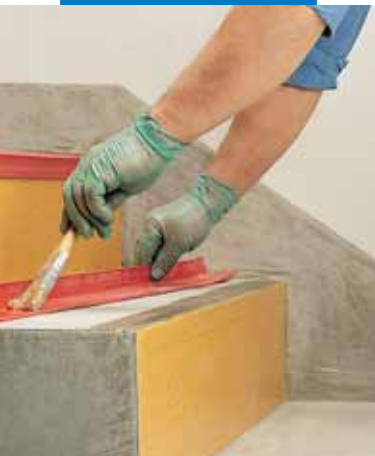
Spreading Adesilex VZ on the backing of a PVC step nosing
