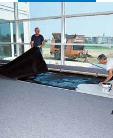
Installing industrial flooring in an electronics company
