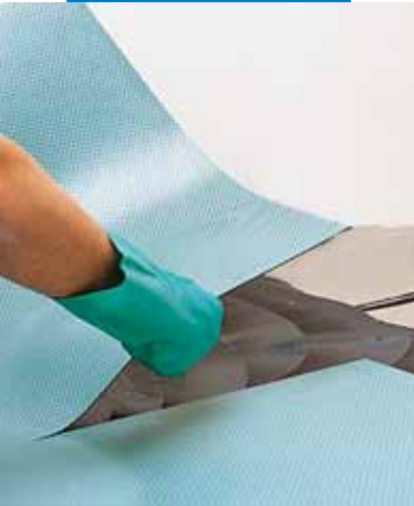
Laying conductive PVC tiles
