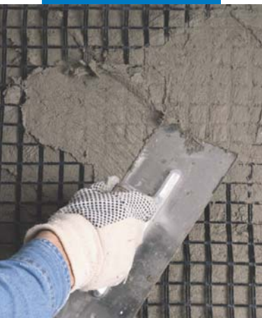
Positioning of Mapegrid G 220
