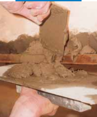
Restoring the front of the concrete slab of a balcony: applying Planitop 400
