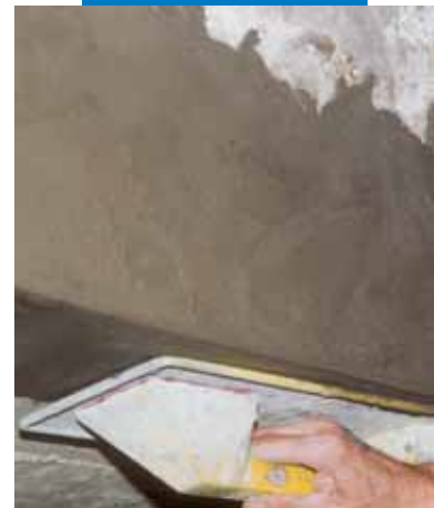
Patch-work of a concrete beam
