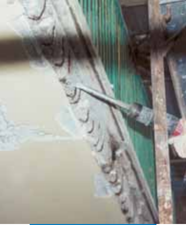
Restoring the front of the concrete slab of a balcony: preparing the substrate
