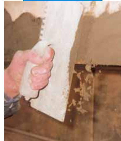
Restoring the front side of the concrete slab of a balcony: finishing
