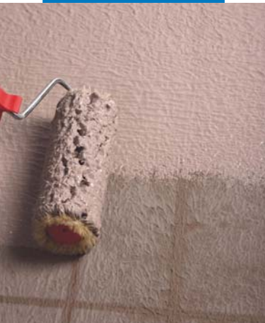
Waterproofing of terraces by roller
