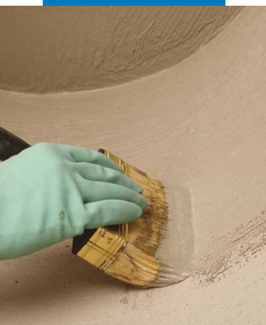
Waterproofing of terraces by brush
