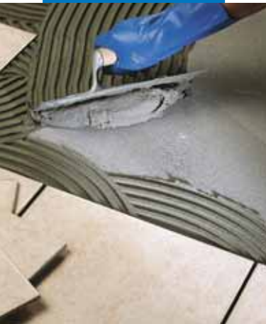
Installation of single-fired tile on floor
