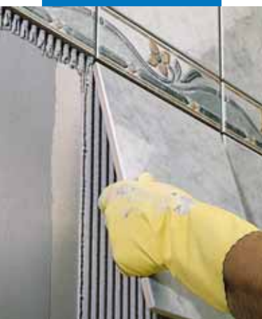
Installation of single-fired tile on wall render
