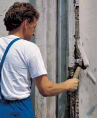
Demolition of degraded concrete
