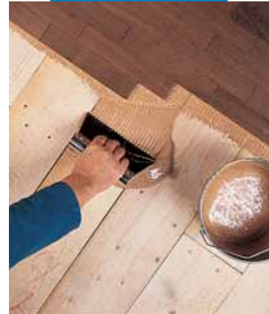
Installing wood strips over floorboards with Lignobond
