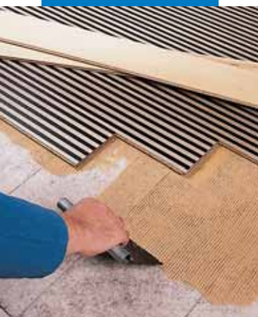
Installing coloured wood strips over existing parquet with Lignobond
