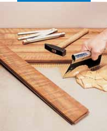
Installing wood strips with Lignobond
