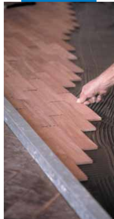
An example of an installation of a wooden floor on existing ceramic tiles with Lignobond
