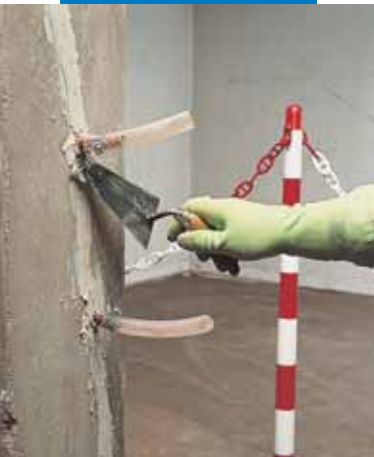
Fixing injection tubes with Adesilex PG1
