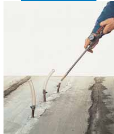
Restoring horizontal structure by injection with Epojet
