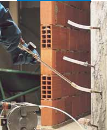
Injecting Epojet to a fissured pillar
