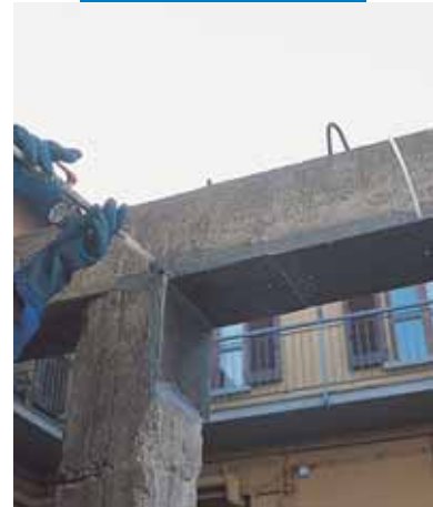
Repairing beam with injection of Epojet
