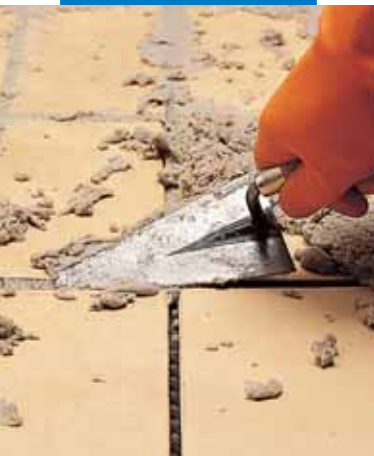
Filling the joints with Kerapoxy SP using a pointing trowel
