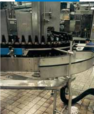
An example of a grouted brewery floor
