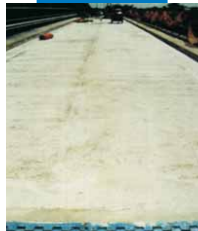
The repaired bridge-deck
