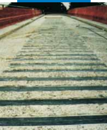
A bridge-deck reinforced with Carboplate
