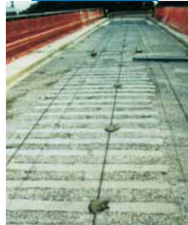
Carboplate covered with Mapegrout BM
