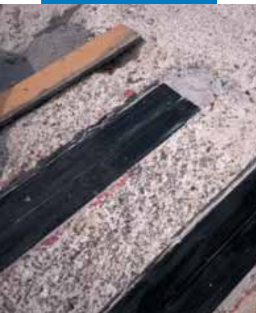
Fixing Carboplate in especially created areas on the substrate
