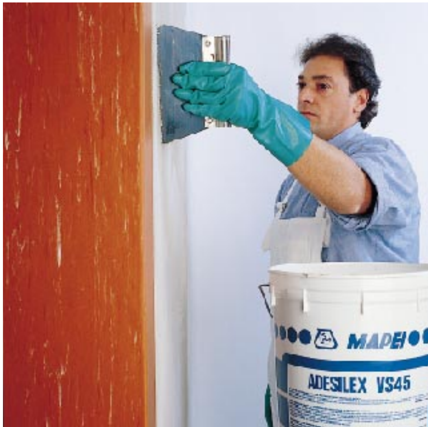
Applying adhesive after turning a corner with a sheet of PVC
