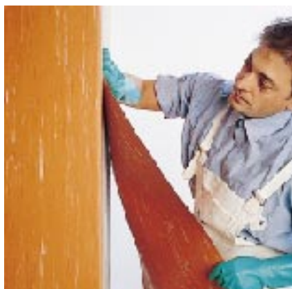
Placing the adjoining sheet
