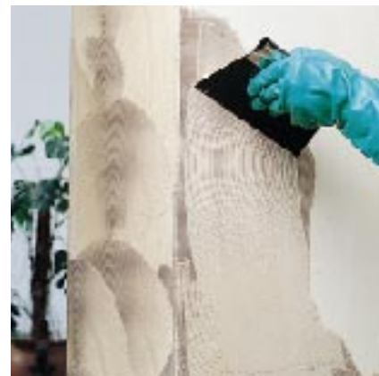
Applying ADESILEX VS45 with n. 1 trowel
