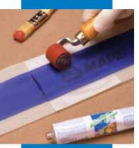
Use a roller to press the joints of the Mapeband strips together
