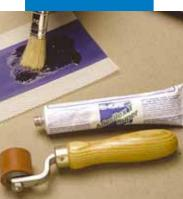
Spread the Adesilex T Super on one of the two strips of Mapeband to be joined
