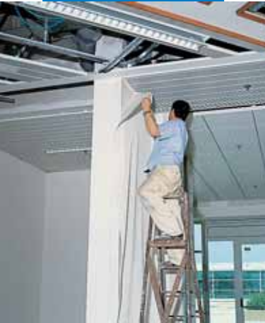
Installation of wall covering in offices
