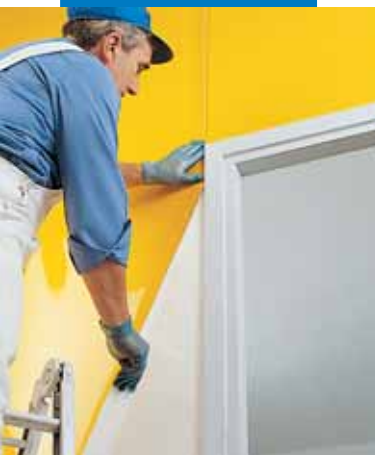
Installing sheets of wall coverings with Adesilex MT32
