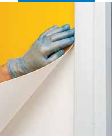
Detail of installation
