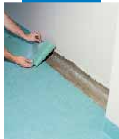
PVC scarting installation
