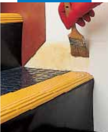
Installing rubber skirting with Adesilex LP
