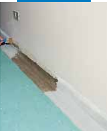
Istituto Tumori - Milan - Installing PVC floor with Adesilex LP
