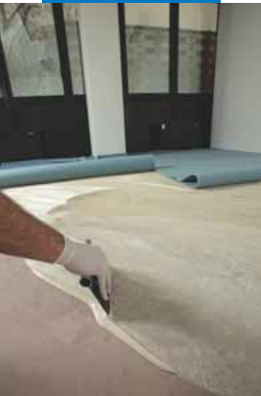
Applying Ultrabond Eco 170
