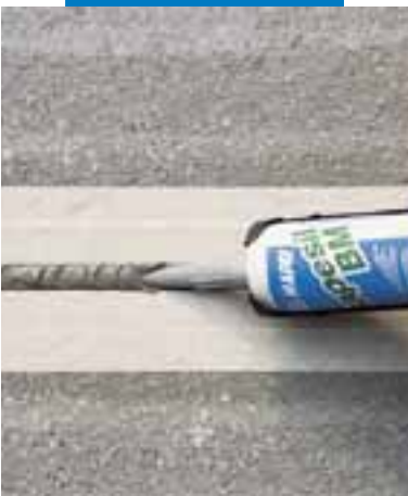
Joint filling with Mapesil BM
