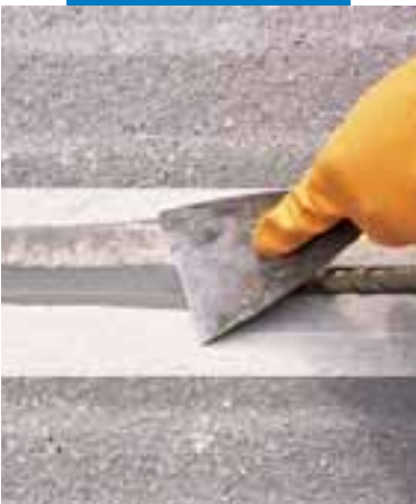
Joint smoothing by removing the excess sealant
