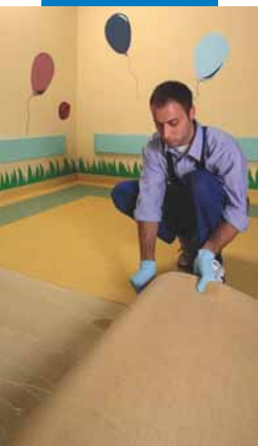
Installing linoleum sheets with natural jute back
