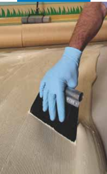
Applying Ultrabond Eco 520
