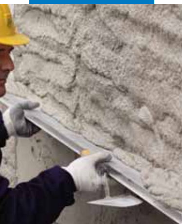
Levelling off the render
