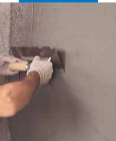
Applying Planitop 540 with a metal trowel
