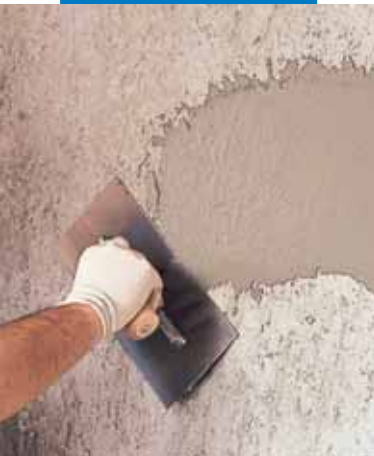
Applying Planitop 540 with a metal trowel
