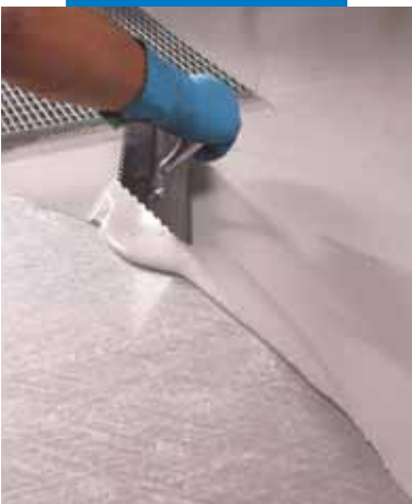
Applying a second layer of Monolastic on Mapetex Sel
