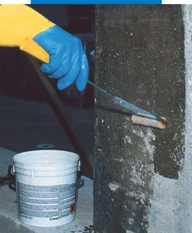
Applying a second coat of MapeWrap Primer 1
