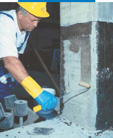
Applying a first coat of MapeWrap Primer 1
