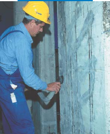
Preparing the substrate
