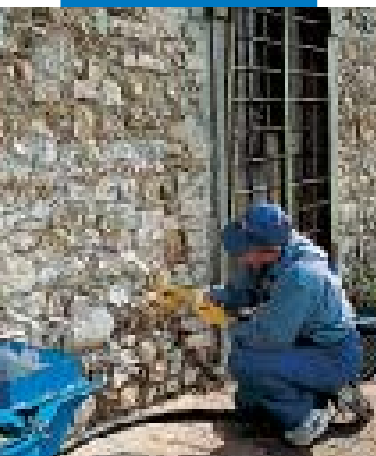
Consolidating injection with Mape-Antique I
