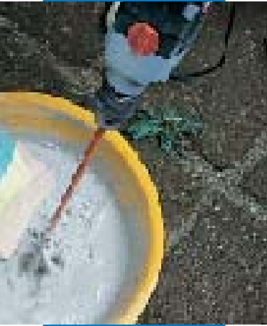
Preparation of the Mape-Antique I slurry
