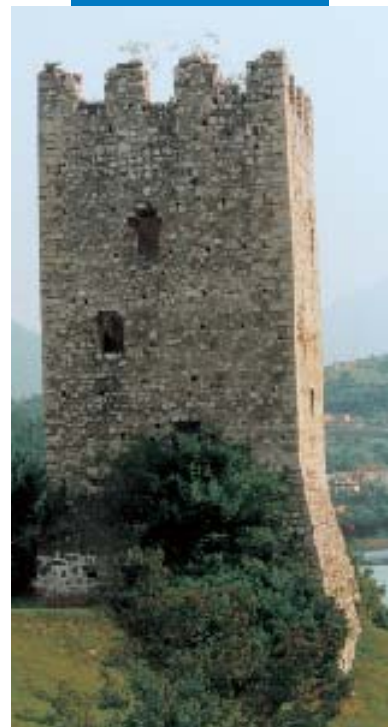
San Floriano tower consolidated with injection of Mape-Antique I
