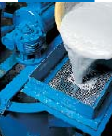
Filling of the injection pump with Mape-Antique I
