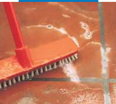
Cleaning with Keranet liquid by polishing brush
