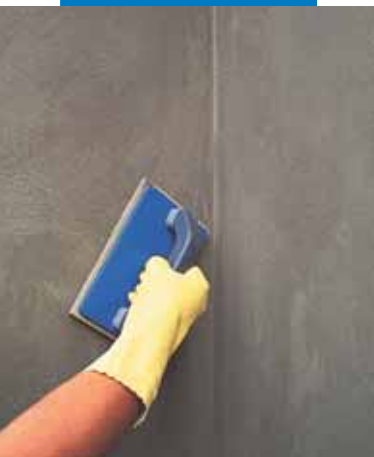
Finishing with sponge float
