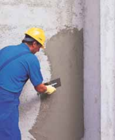
Application by trowel
