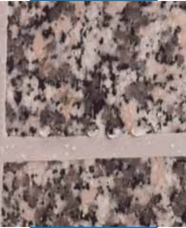
Sealing an external stone dressing
