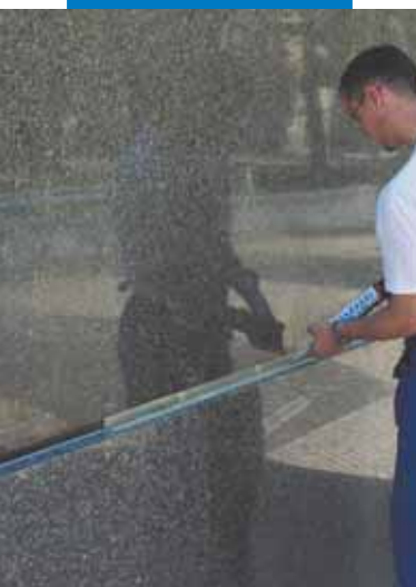
Sealing a façade joint with Mapesil LM
