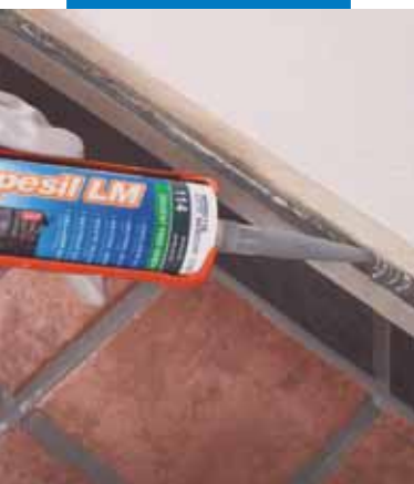
Sealing an internal stone dressing
