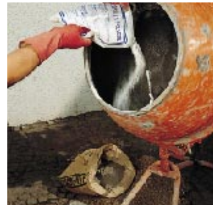
Preparing waterproof mortar admixed with IDROSILEX POWDER
