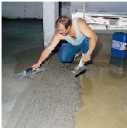
Screeding with mortar admixed with IDROSILEX LIQUID
