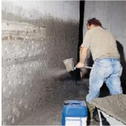
Spraying on the first coat of mortar admixed with IDROSILEX LIQUID
