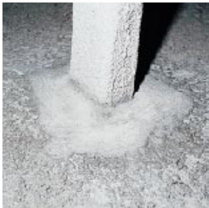
Column waterproofed with IDROSILEX
