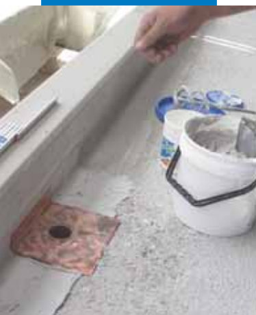
Laying a copper neck-flange and drain spout
