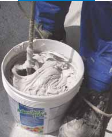
Preparing the mix
