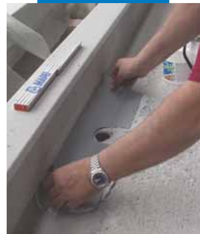
Laying flexible hypalon brace
