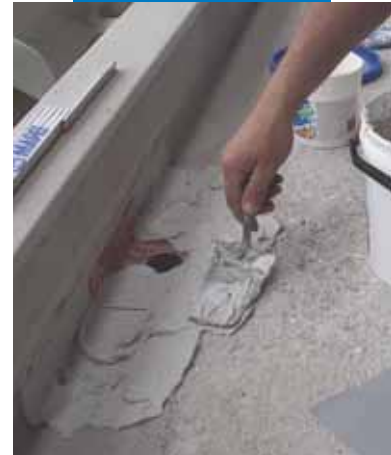
Subsequent smoothing with Adesilex PG4
