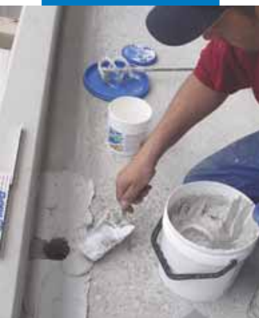
Applying Adesilex PG4 with a trowel
