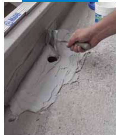
Final covering with Adesilex PG4
