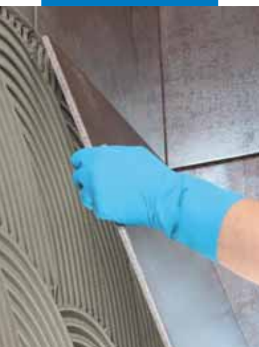
Laying large-sized tiles on walls
