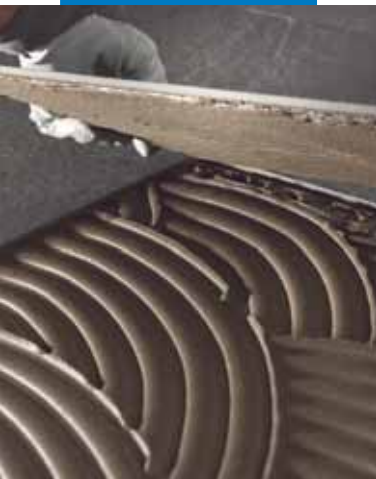
Installing thin porcelain tile on floor
