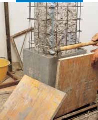
Removing wooden formwork
