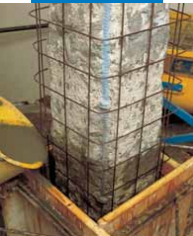
Pouring into a formwork
