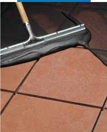
Grouting a terracotta tile floor with float
