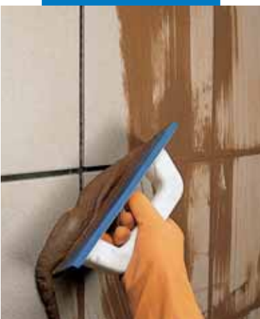
Grouting an external wall with a float
