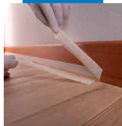
Removing the protective paper tape
