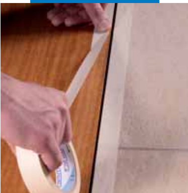
Protective preparation of the sealing of the joint
