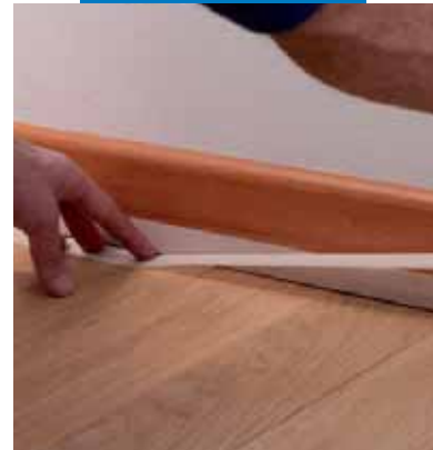
Protective preparation of the sealing of the joint
