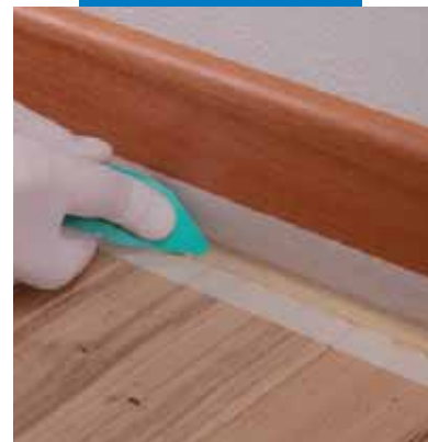
Finishing off the surface
