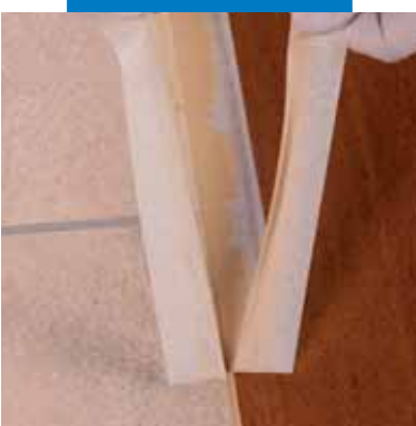
Removing the protective paper tape
