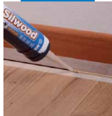
Filling the joint
