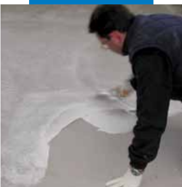
Primer MF thickened with Additix PE
